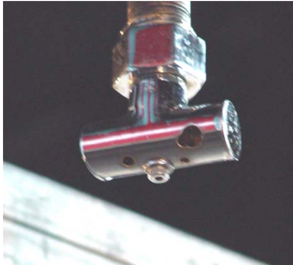
Figure 3. CAF Delivery Nozzle
